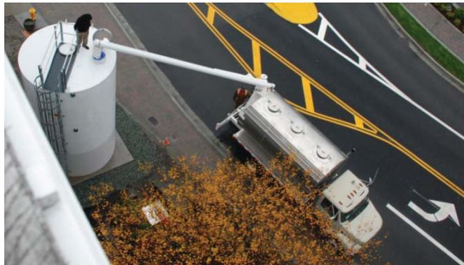
Wood pellet fuel is delivered to the storage silo
