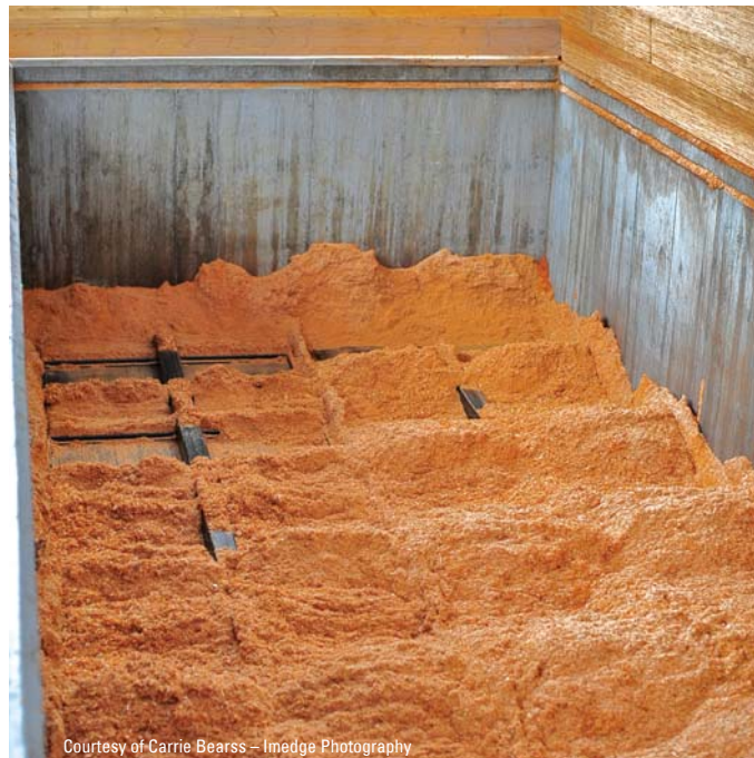
Courtesy of Carrie Bearss – Imedge Photography Fully-automatic feed system ensures consistent fuel supply and reliable operation
