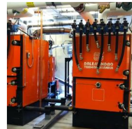
A biomass thermal system can provide hot air, water, and process heat
